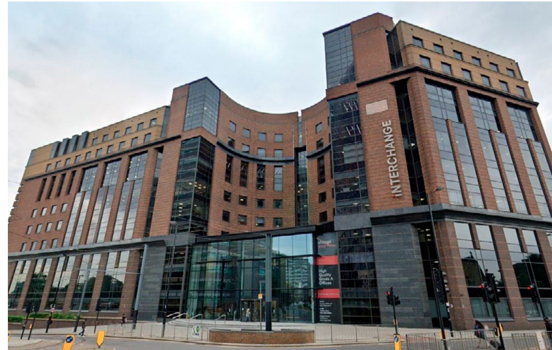
Interchange House, 81–85 Station Road, Croydon Canmoor Asset Management/Tristan Capital Partners
